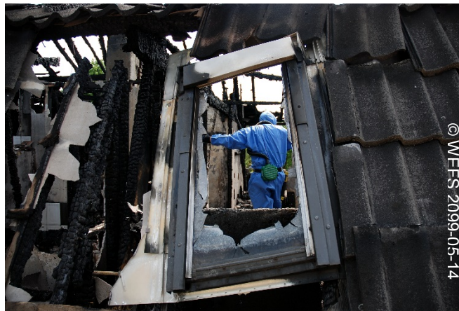
Asbestos removal work after a fire
